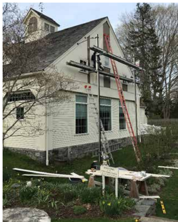
Archives second-floor window installation
