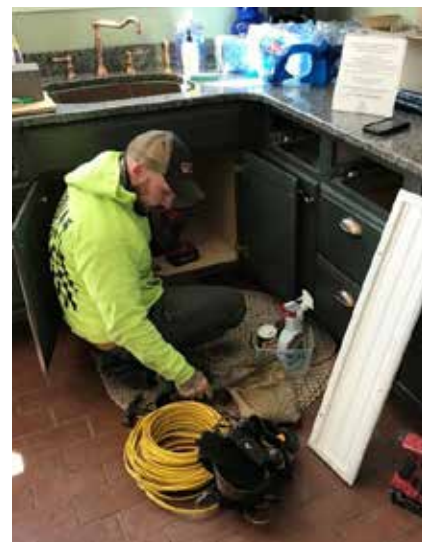
Majestic Electric employee (Josh) installing photo electric circuit
