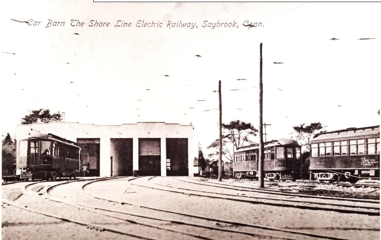
(Above and below): The trolley car-barn on Ford Drive, which still exists, photographed from the old overpass, which no longer exists.
