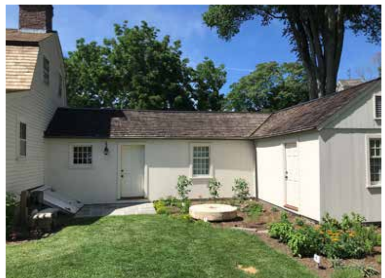
Hart House Gallery South Siding and Garden Project, June 2024
