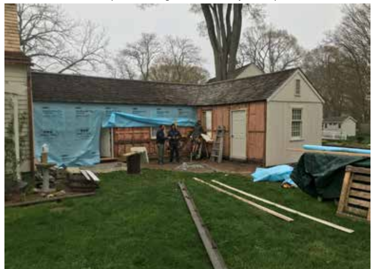
Hart House Gallery South Siding and Garden Project, May 2024 Photo
